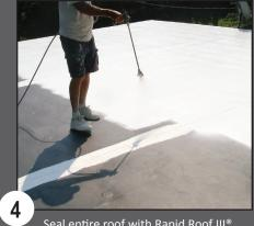
Seal entire roof with Rapid Roof III® Top Coat or Equinox<sup>®</sup> Top Coat
