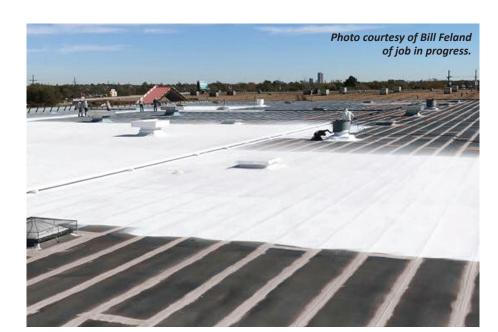
"I like the versatility, strength, and waterproofing capabilities of the Membrane Coating System. The available 10-year warranty\* gives both my customers and I peace of mind. The high-quality Spunflex<sup>®</sup> fabric used in this system is flexible and easy to work with. Due to coastal wind uplift and potential hurricanes, having a seamless commercial roofing system is a must here in south Florida!"
