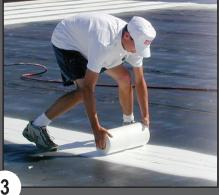
einforce seams with Spunflex<sup>®</sup> embedded in Rapid Roof III® Base Coat or Equinox<sup>®</sup> Base Coat.
