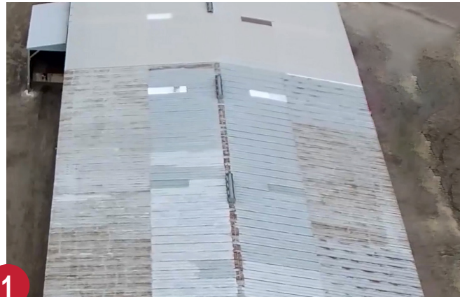
Rusty metal roof prior to restoration work.
