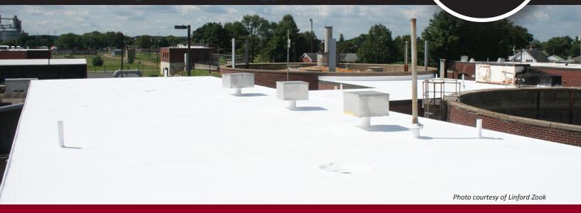
Highly reflective "cool" roofs are having their day in the sun. During the warmest weather, studies have indicated that they lower roof temperatures by up to 40% and decrease the amount of heat transferred into a building's interior. That helps reduce energy needs for cooling, and using less energy not only saves money, it also reduces the amount of pollutants released into the atmosphere. Conklin Roofing Systems meet the very highest standards for energy efficiency.
